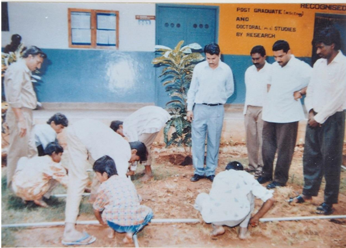
Coupling pipes during a plumbing training
