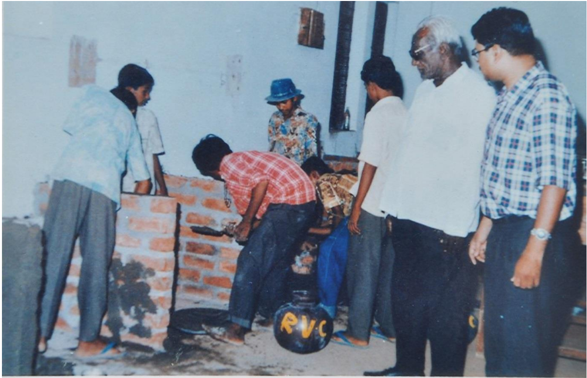
Guiding the burnt brick masonry work in CM 1:6
